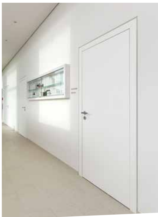
Elemento insonorizador / Soundproofing element Puerta, bastidor y pared empotrados, ranura ancha giratoria Flush door, frame and wall, shadow groove all around
